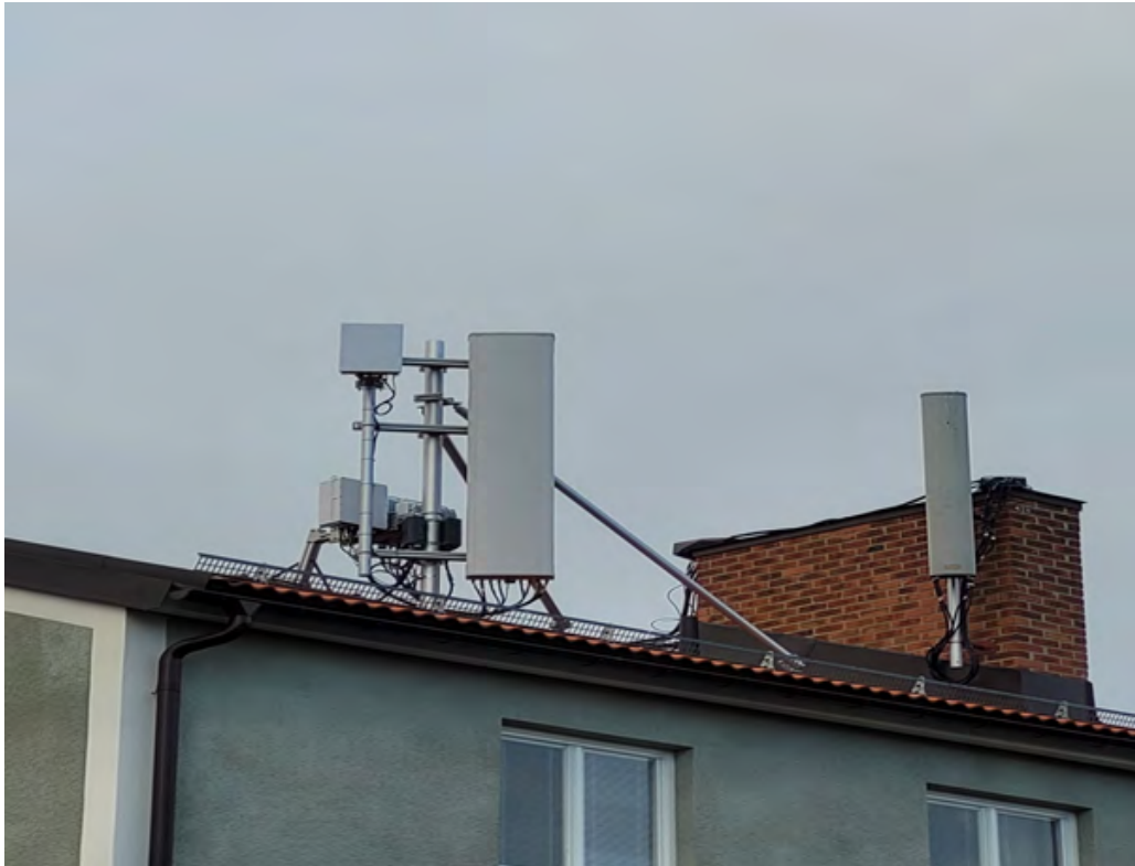
Figure 3: 5G base station on the roof of a three floor building located 60 meters from the study apartment. Initial figure after the 5G installation showing the previous base station attached to the chimney
